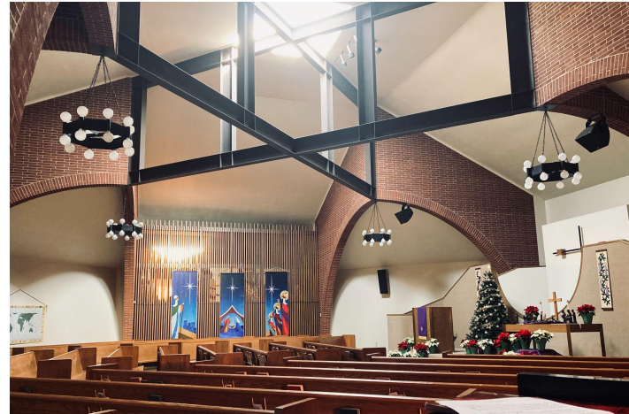
Nave: Skylight above steel frame
