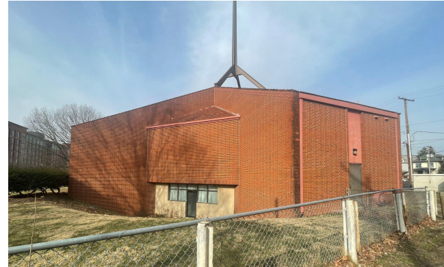
East side (entrance to basement and stairwell)
