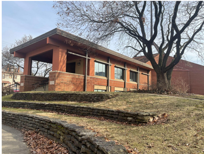
West side (main entrance)
