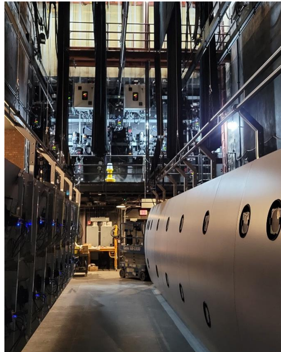
Rigging wall after the renovation.
