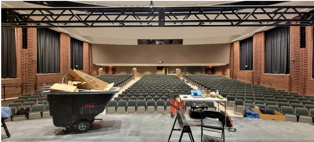
Auditorium after the renovation.
