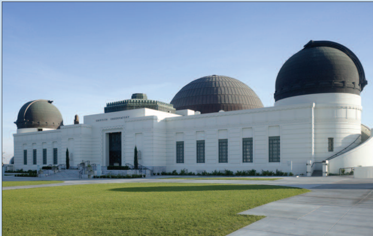
PHOTO: TIM GRIFFITH
