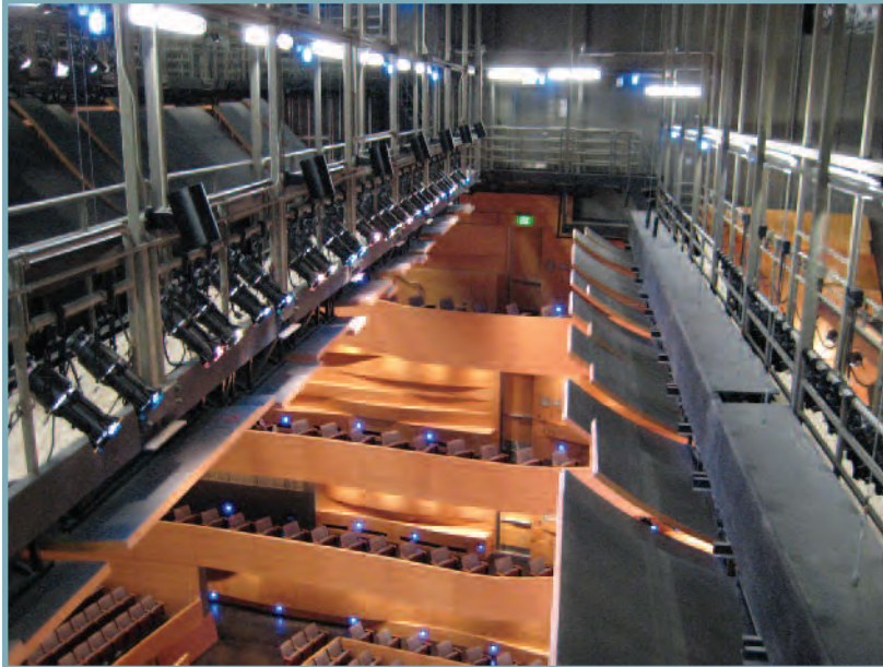
Drapes can be raised from within these catwalk enclosures to provide sound absorption.
