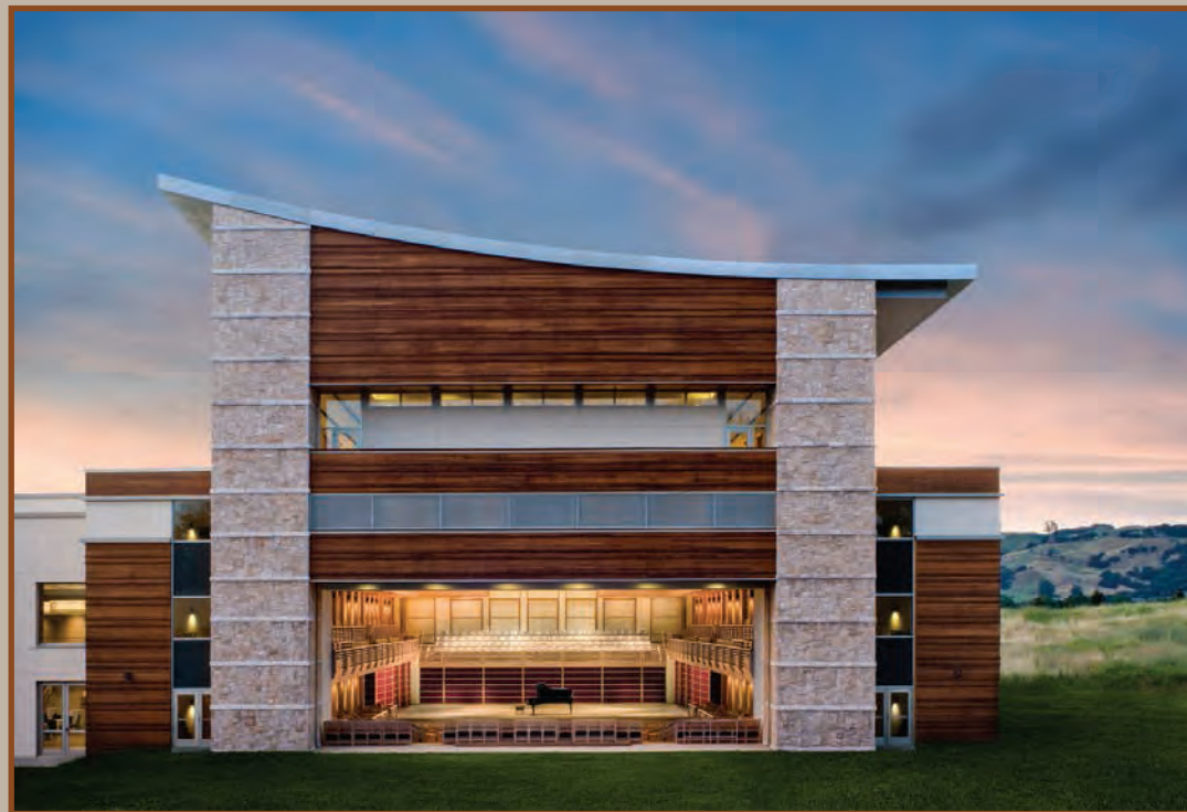
The exterior of the Sanford I. Weill Hall, with the rear wall of the auditorium open to the lawn.
